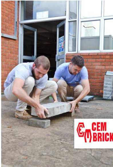
Bond test for flexible mortar mix – WIL students Hendrik (left) and Johno
